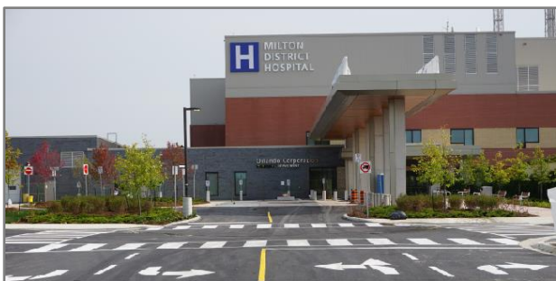
Milton District Hospital
